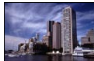
Photo Courtesy of MOTT
